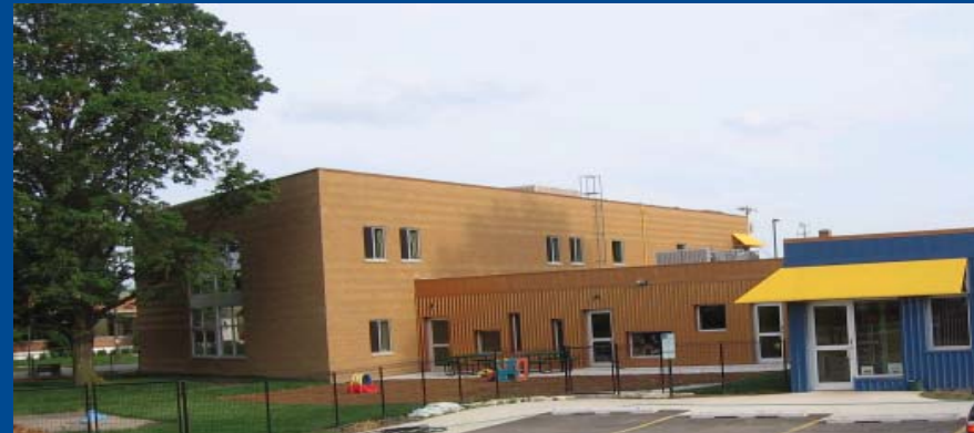
The renovated Family Center facility.
