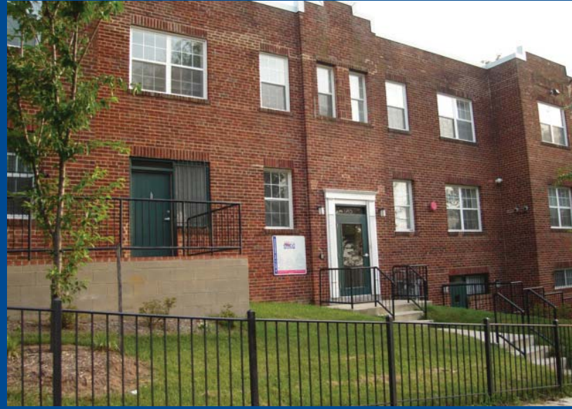
The renovated Good Hope House in Washington, DC (above). The families in residence at Good Hope are stable in their recovery programs and are moving towards the foundational goals of increasing household income, maintaining sobriety and attaining permanent housing.
